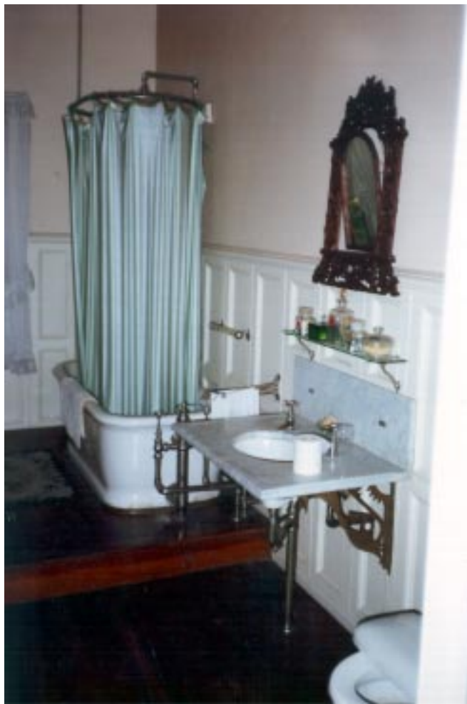
Bathroom as pictured in a photograph taken before the 1985 fire damaged the room considerably. The blueboard system should be used for the wall repair and the paneled wainscoting
