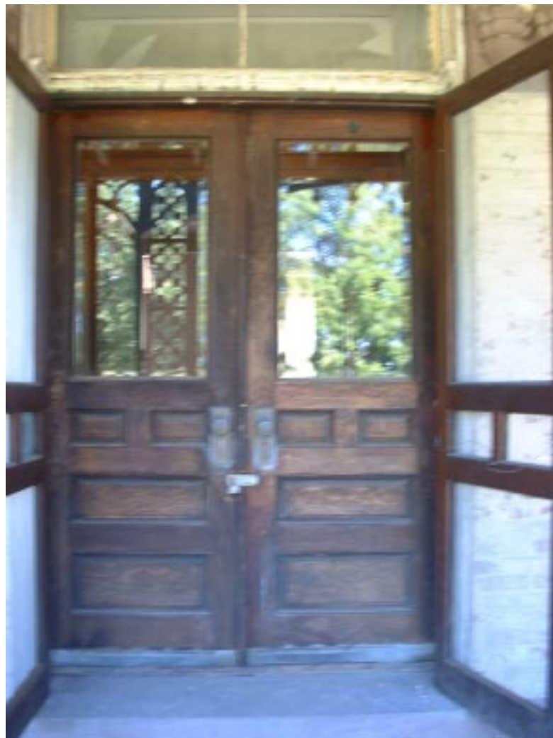
The main entrance to Maple Grove was re-configured in 1891. Paneled doors with beveled glass open into a small vestibule and the house is entered through another set of paneled doors. Note the transom light above the doors.
