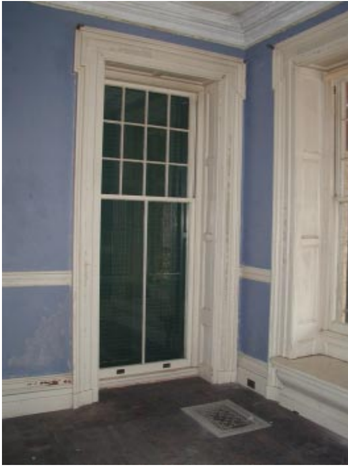
Right: 1990s photograph of southwest corner of Drawing Room. Note the paneled window jambs, the dog-ear window architraves and the multi-lite upper sash in the windows. Visible in the lower right of the photographs the floor register near the corner that provided heat to the room after 1891. The window sash measure 50-1/2" x 45" (lower) and 50-1/2" x 43" (upper) for the west window and 64-1/2" x 40" (lower) and 43" x 40" (upper).
