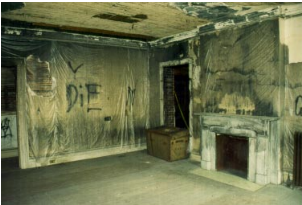
The southeast corner of Mrs. Kinkead's Morning Room. The door on the left leads to the Passage and the door in the middle led, at one time, to a dressing room. Note the band of block parquet flooring at the perimeter of the room, the marble chimneypiece and the tile hearth.
