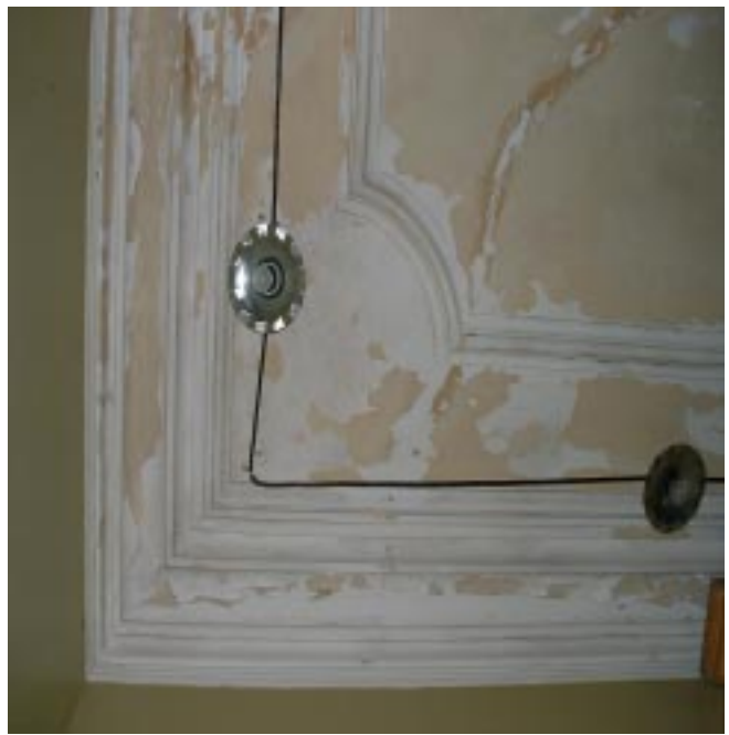
Detail of the Greek Revival cornice northwest corner of the Grandparent's Parlor. Note the deep cove between the two outside bands and the bolection molding with convex curves marking the corners.
