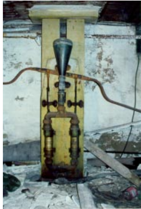
Water pump installed in the late 19 th century. Note the unique double-arm pump mechanism.
