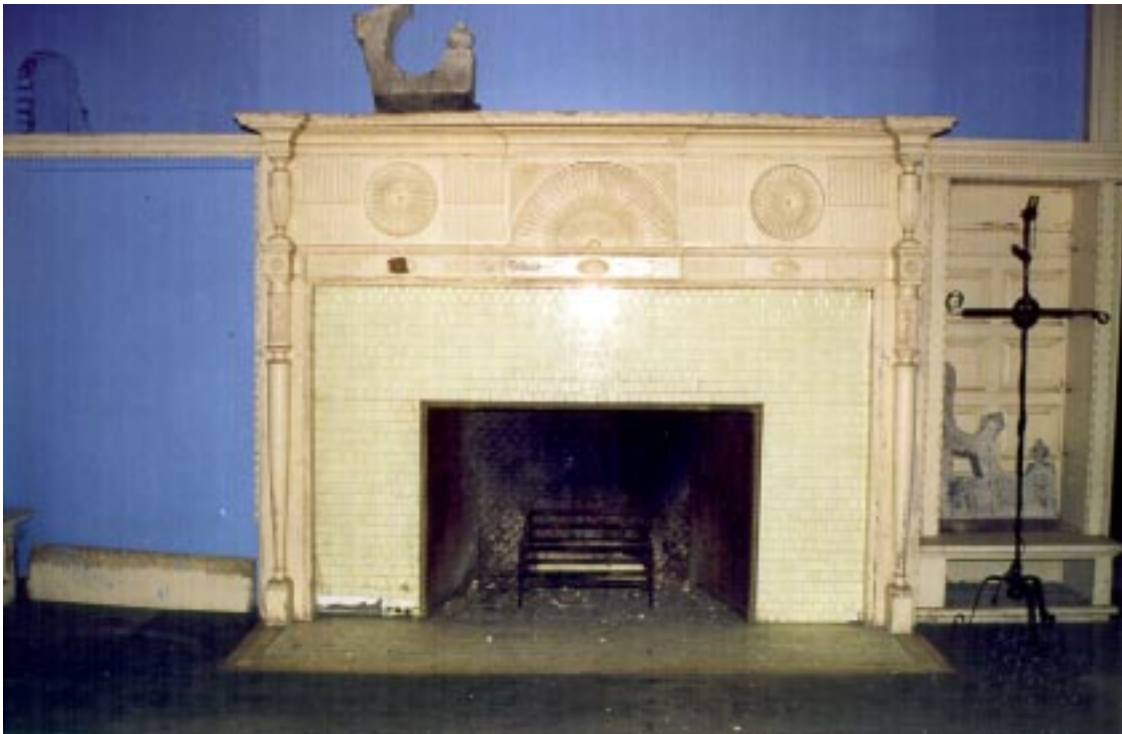
The fireplace dominates the living hall space of the Library. The delicately carved chimneypiece extends inches above the line of the dado rail. Tapered cylindrical columns rest on small plinth block and extend up to the carved entablature. A broad frieze panel incorporates roundels and a fan pattern as its focal elements with a dentilled cornice. Creamy yellow glazed tiled, 2-1/2” square, are used for the slips and hearth. The hearth is trimmed with a band of 1/2”x 4-1/4” reddish gold tiles and a second band of 2-1/4”x4-1/4” yellow tiles with a floral pattern and is flush with the parquet floor. A cast-iron liner was inserted into the firebox.
