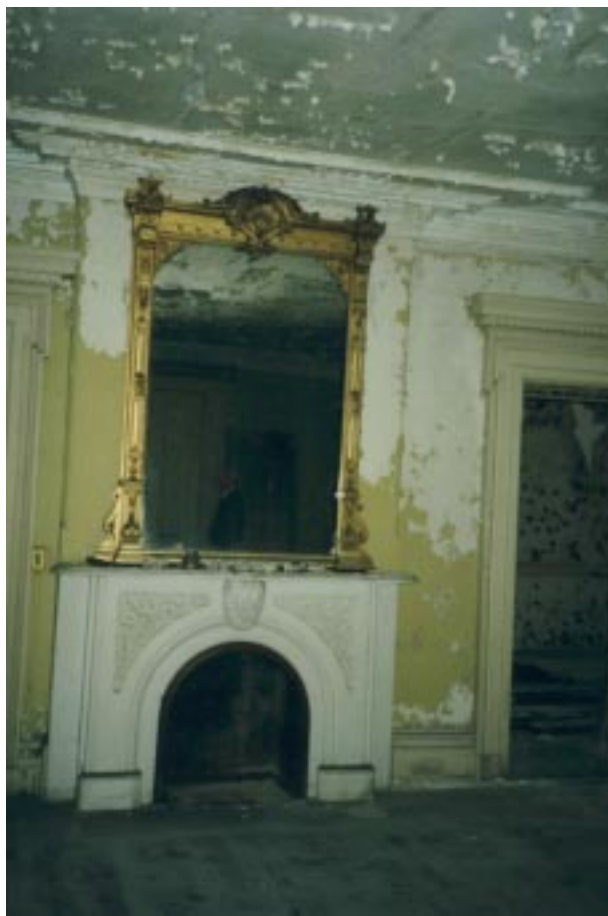
The white marble chimneypiece in the Grandparent's Parlor is complimented by a gilded Renaissance Revival mirror. The fireplace hearth is a darker marble, set flush with the floor. The mantelshelf is approximately 4' high.
