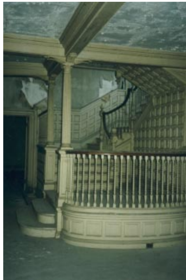
The curved landing of the staircase provides a small seating area that overlooks the Library. Note the sweep of the handrails from the landing, the wainscotting that follows the stairs, the fluted columns and twist-turned balusters. The walls above the dado were originally papered as seen on the north wall pictured here.
