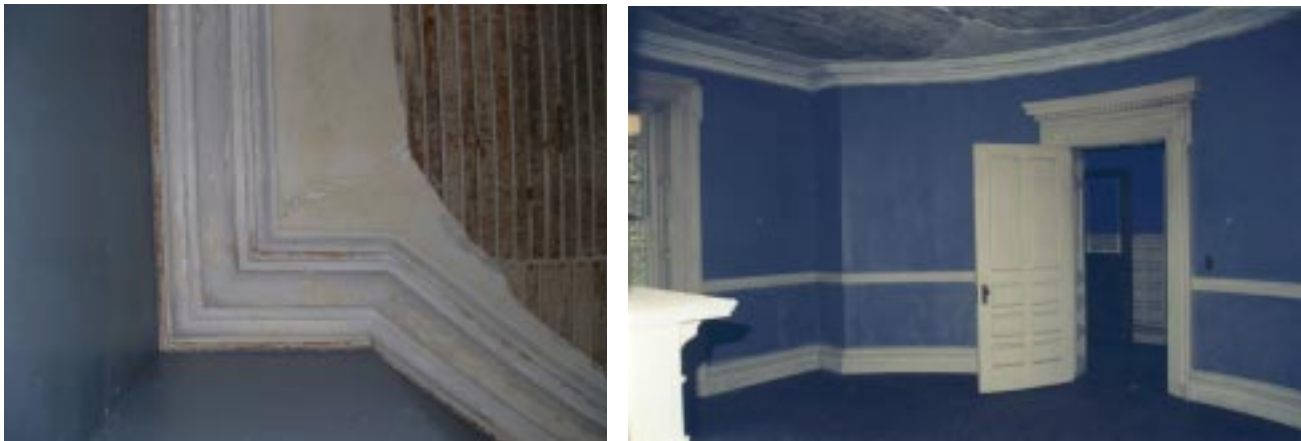
Right: Detail of the cornice molding in the northwest corner of the Drawing Room. Note the beginning of the graceful curve of the wall and the deep cove between the two bands. Left: The northwest corner of the Drawing Room. The curve of the wall allows for a small closet in the Vestibule. Note the dog-ear architraves surrounding the doors and windows and the Colonial Revival cornice additions with dentils applied in 1891.
