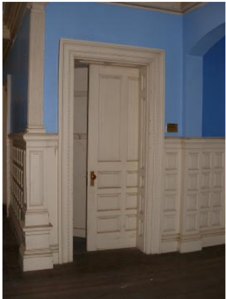
Pocket door at the end of the Passage opens onto a closet with a curved wall. The wainscot runs along all the walls of the Library and Hall as well as the Passage. Note the corner column is fluted above the dado rail. The door architrave is the same as that in the Vestibule.
