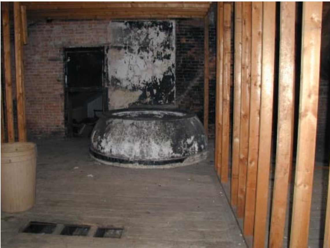
At the center of the photograph is the laylight structure, which is made of plaster and lath. To the left of the shell is the entrance to the trunk room. The cistern is located directly above the 1891 bathroom in the southeast corner of the main block.
